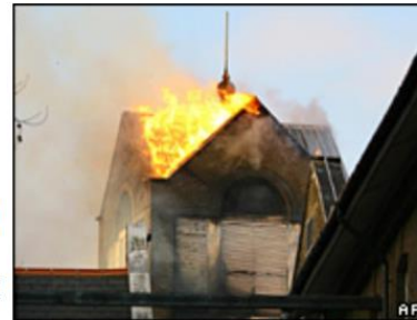
The fire has destroyed much of the top floor
