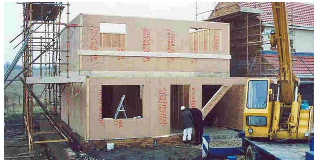
**SIPs – structural insulation panels**
